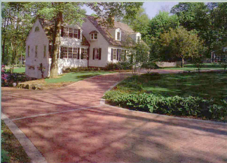
Dyes and surface patterning belie that this driveway is essentially a concrete slab.
