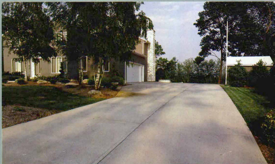
Properly detailed concrete is extremely durable.
