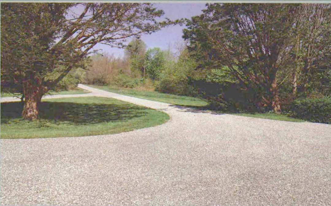
Gravel bonded to an asphalt base adds a wearing layer, making a more durable finish.
