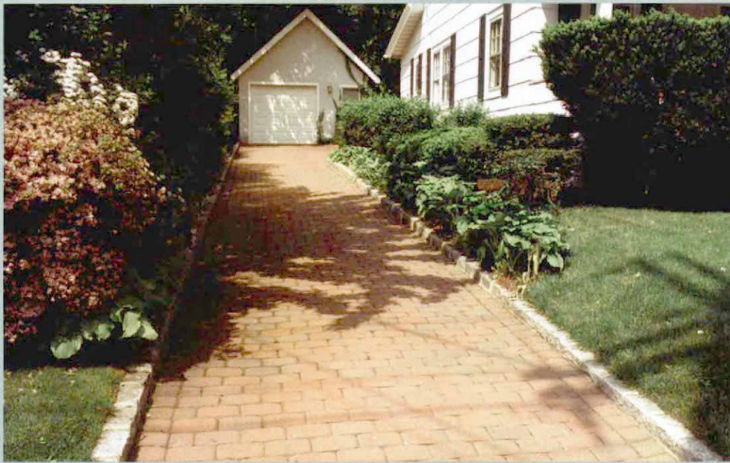
Another form of concrete, precast pavers, come in a variety of shapes.
