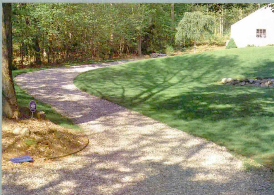
Edging keeps most of this driveway's gravel off the lawn.
